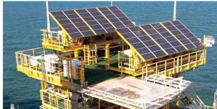
Cloud Notify has already yielded its first results. In Oman, TSS has a hybrid solar power system which is supported by diesel generators. A short circuit occurred due to a faulty connection after some maintenance activities were performed. "We immediately received an alarm," Sébastien says.
